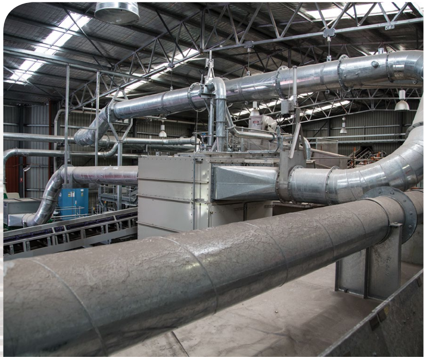
Point source extraction ducts and piping for capture and movement of odorous air into a plant Odour Management System (OMS) for treatment.
