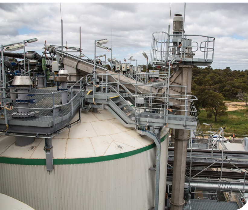
DiCOM™ vessel roof structure showing vertical lift conveyor and vessel loading conveyor.
