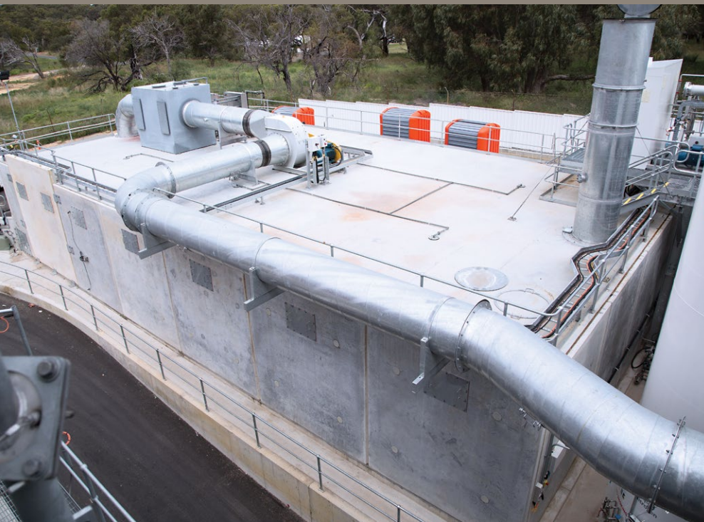
Biofilter based OMS for onsite treatment of ventilation air and gases.
