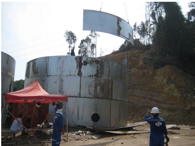
Photographs; Construction activities at the Lubuk Mandi Tailings Processing Plant site in Malaysia. Top, welding of panels for tailings surge tanks, bottom left lifting a panel into position, bottom right tailings plant site vista.
