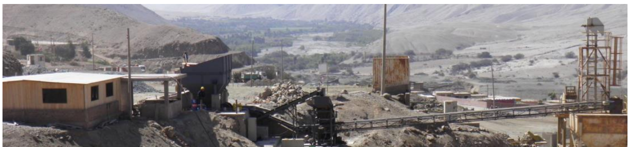
Picture 1: Minera Gold Site office at the San Santiago plant overlooking the ROM Pad and new primary and cone crushing circuits.
