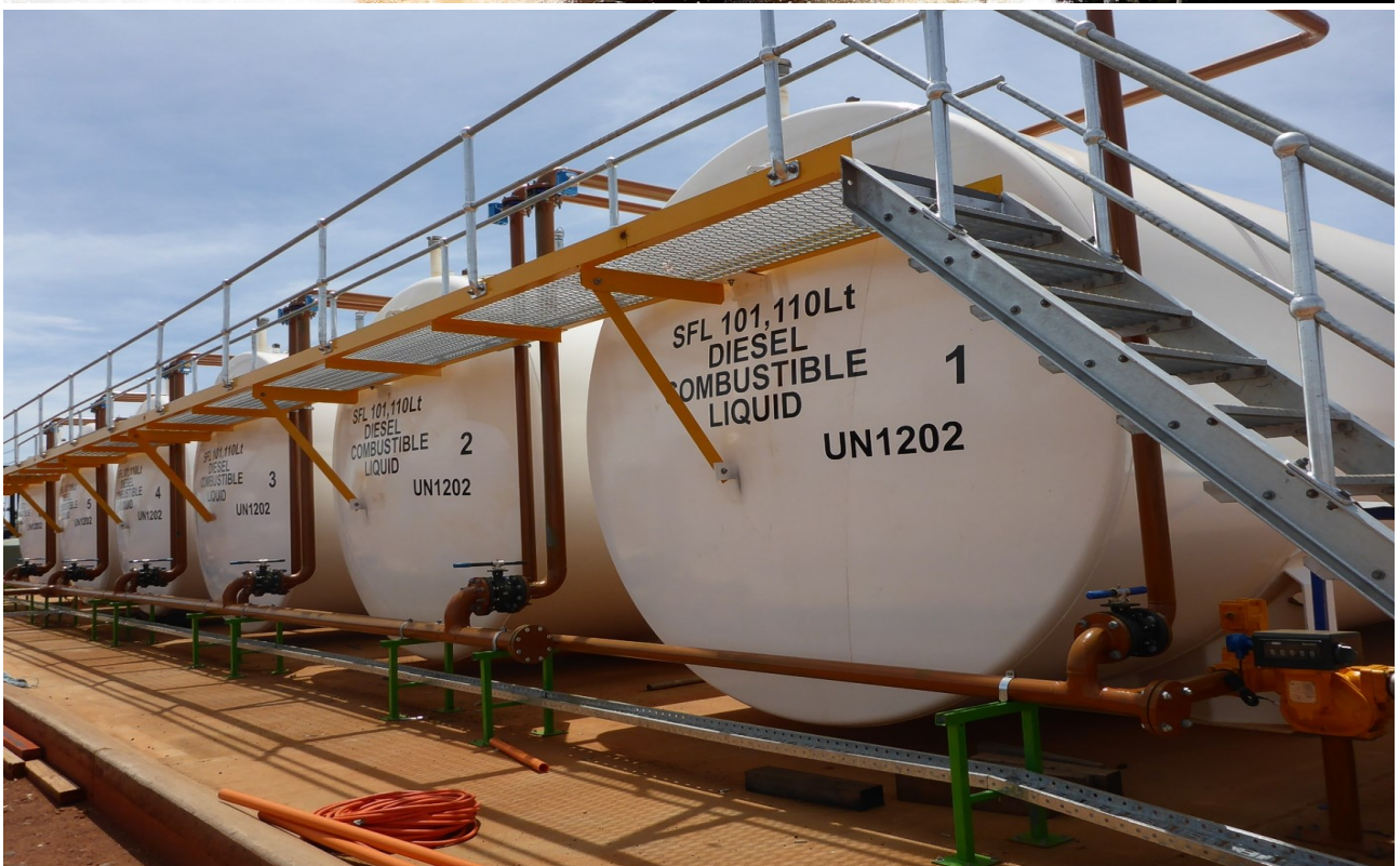
Figure 4: Wet season rains are helping to fill the Water Storage Facility (WSF), and; Process Plant Fuel Farm is complete and has a storage capacity of 600,000 litres.
