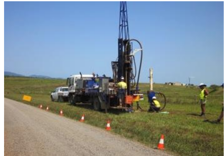
Aircore drilling underway at South Johnstone Project
