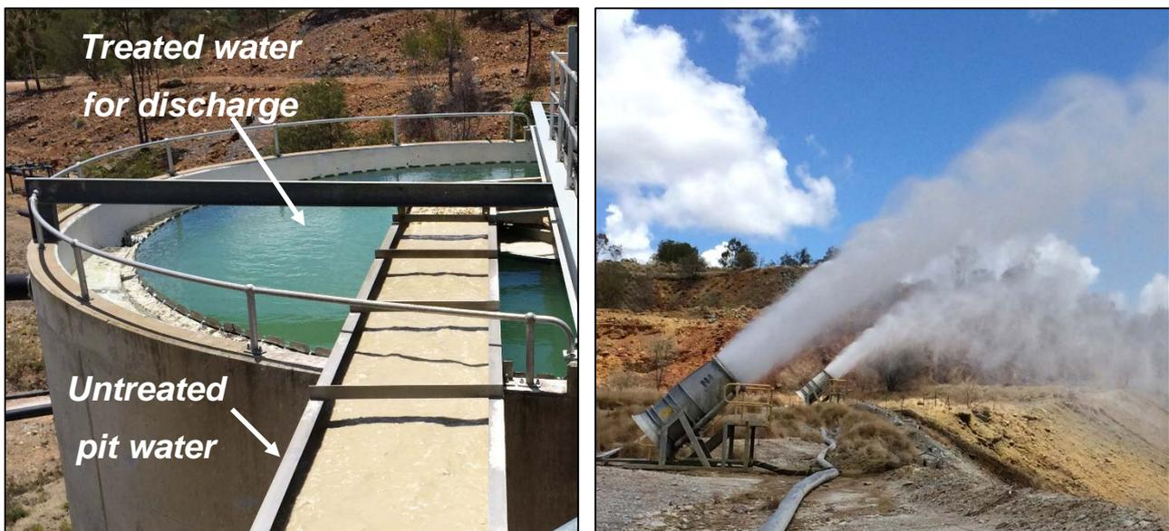
**Figure 5: Operating water treatment plant and evaporators at the Mount Morgan Mine**
