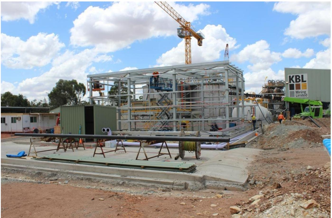
*Photograph 1. Cyanide unloading pad, and CIL gold room construction*
