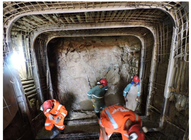
Figure 3. Working face at the end of the Cascavel Incline Shaft. Note the steel, mesh and timber support used to ensure a safe working environment and the long term viability of the main haulage route for ore coming from underground.
