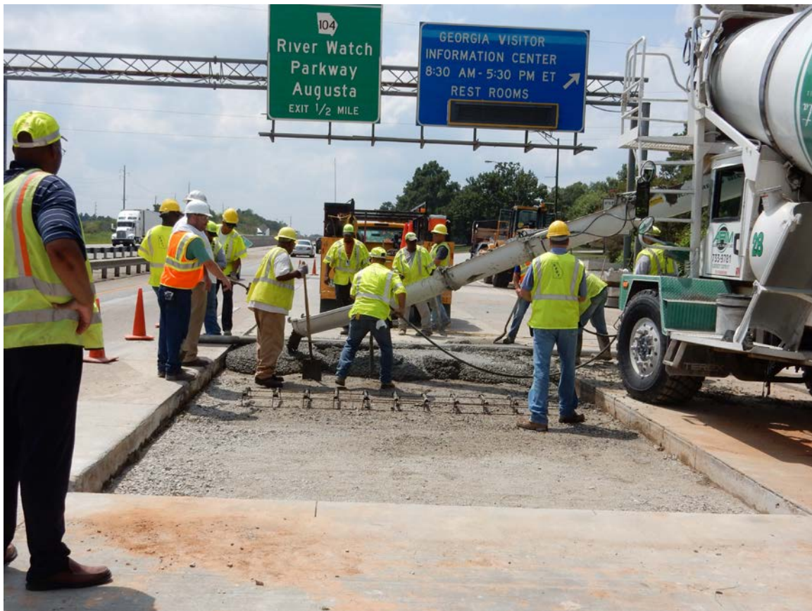
Figure 1 Second Field Trial of EdenCrete™ being Undertaken On I-20
