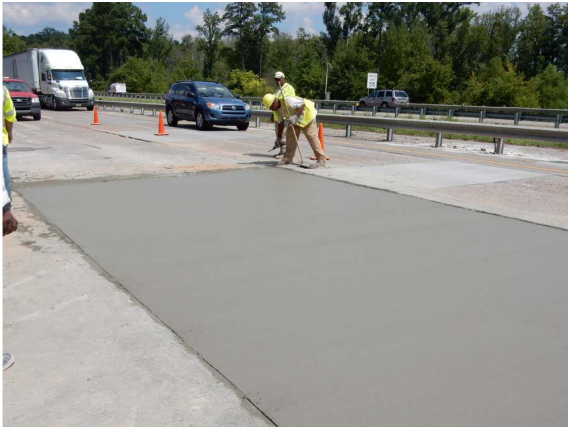
Figure 2 Second Field Trial of EdenCrete™ being Undertaken On I-20
