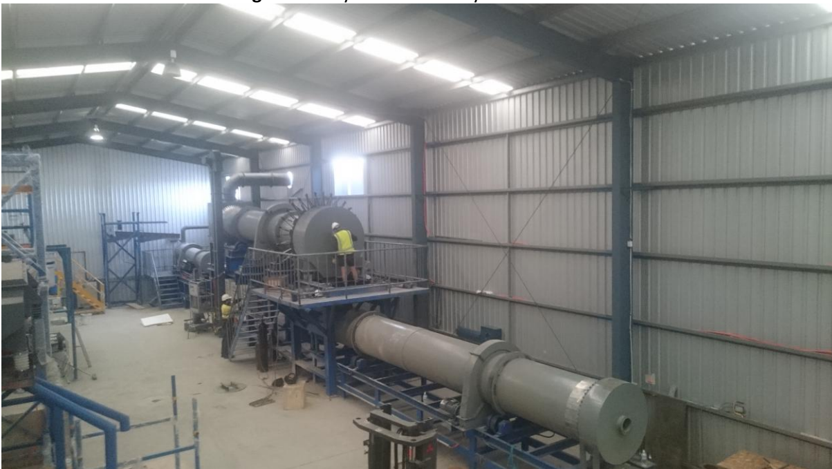
Image 2: Construction team completing refractory of primary sintering kiln.
