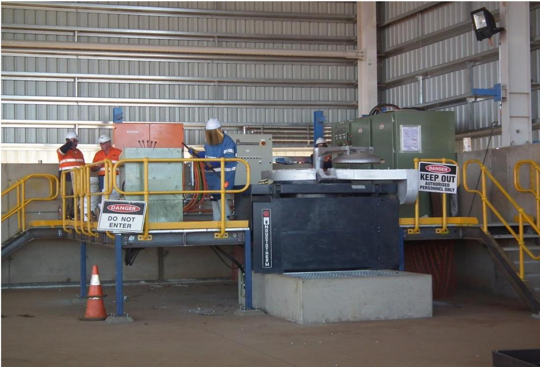
The casting plant and ancillary equipment, including a 1Mw Power station was installed and operational within 3 months of arriving on site. This was installed by CuDeco engineers, independent of the processing plants principal contractor, Sinosteel Equipment and Engineering Co Ltd.
