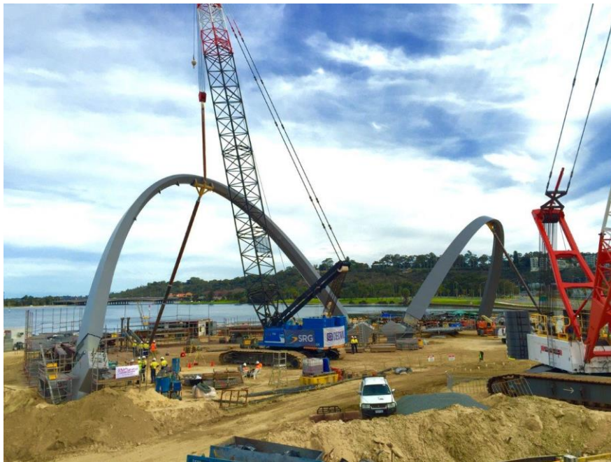
Above: the second arch is lifted into place for the Elizabeth Quay Pedestrian and Cyclist Bridge project
