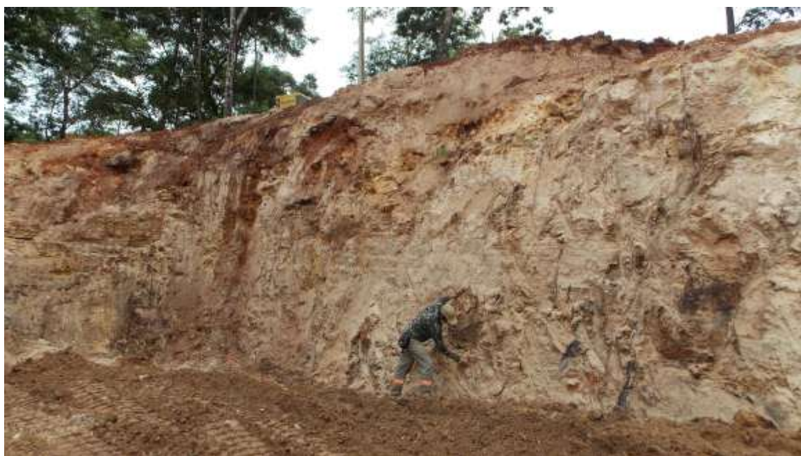
Figure 1. The area of the Cascavel Portal being prepared for the development of the incline shaft.
