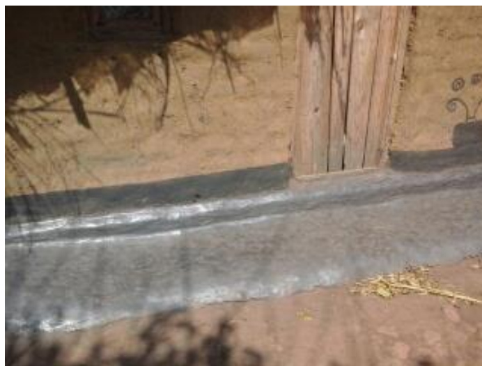
Figure 3. “Chiziro” paint made from locally sourced, purified high-grade graphite on a hut in the Lifidzi area
