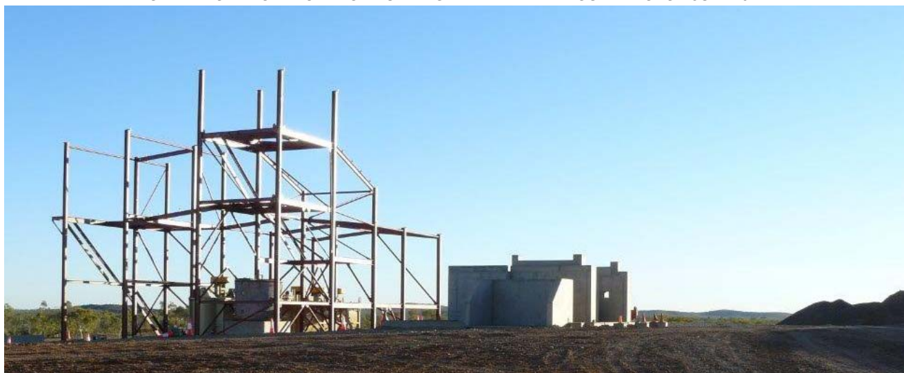
STEEL WORK FOR FLOTATION BUILDING AND BALL MILL FOUNDATIONS – JULY 2014
