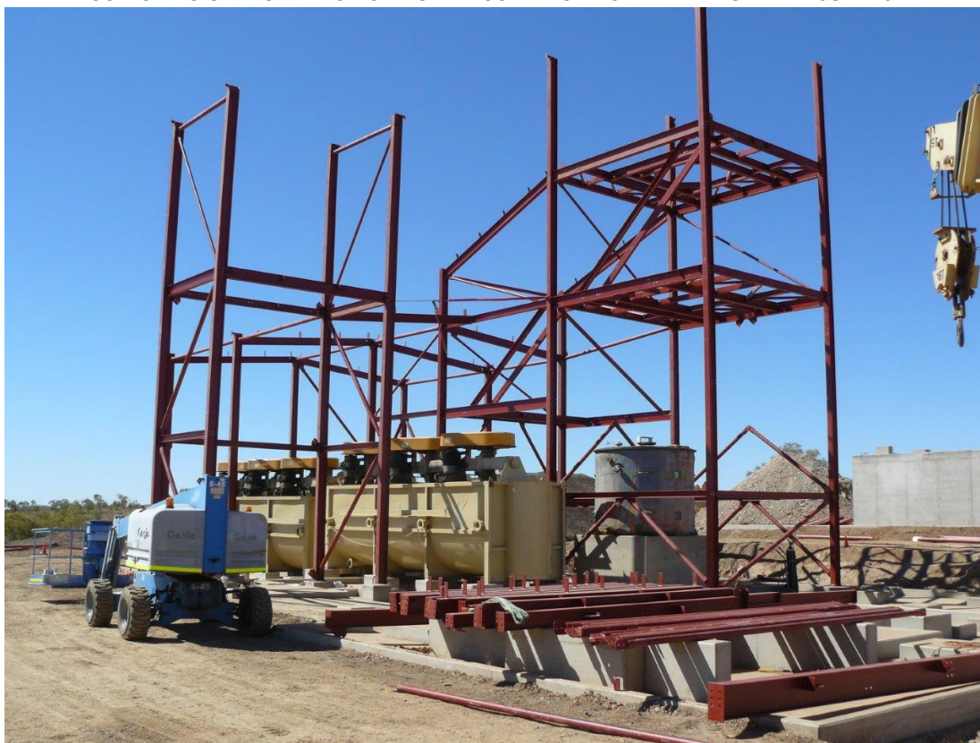
POSITIONING OF FLOTATION CELLS AND CONDITIONING TANK AT LORENA – JULY 2014
